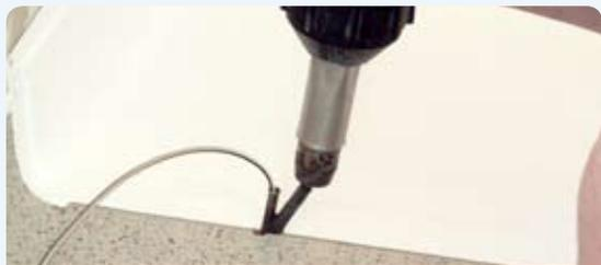
Hot seam weld vinyl flooring directly to the Eagle TWO's TRUESEAL2 profile.
